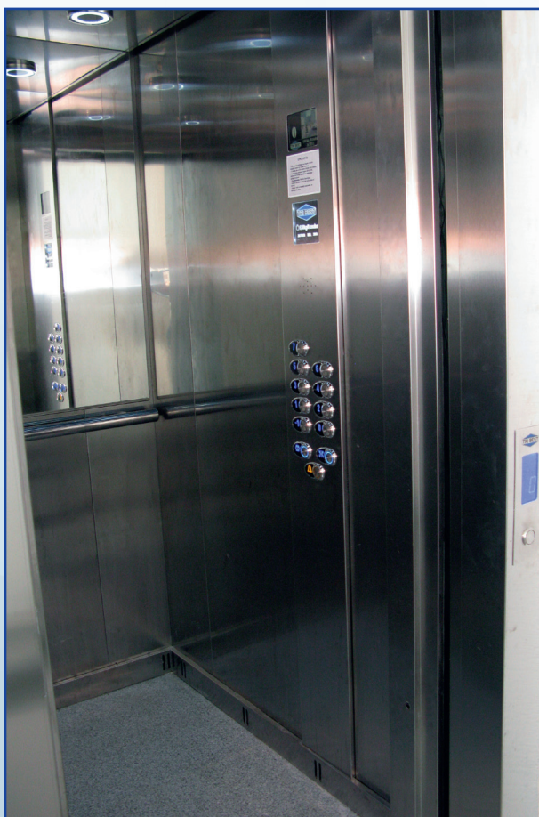
Zidovi inox, pod kamen, strop inox Inox walls, Stone floor, Inox ceiling Wände Inox, Fussboden Stein, Decke Inox
