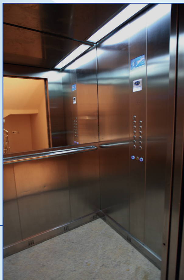
Zidovi inox, pod kamen, strop inox Inox walls, Stone floor, Inox ceiling Wände Inox, Fussboden Stein, Decke Inox
