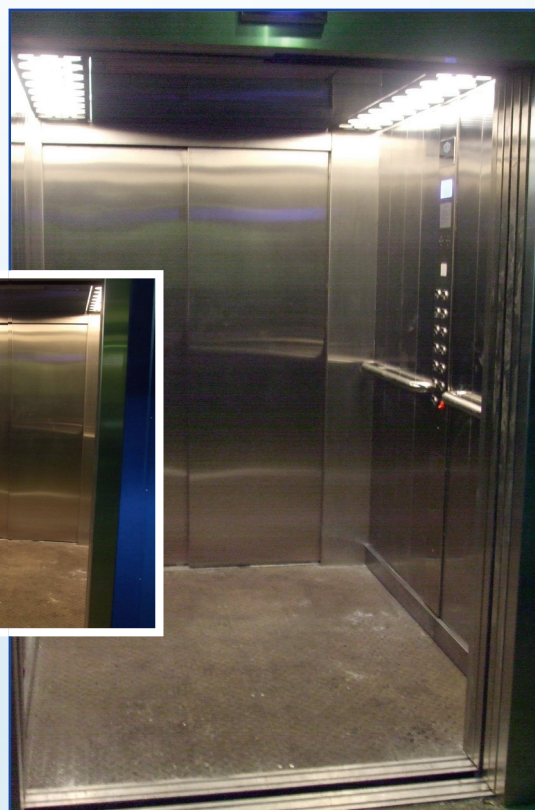
Zidovi inox, pod guma, strop inox Inox walls, Rubber floor, Inox ceiling Wände Inox, Fussboden Gummi, Decke Inox
